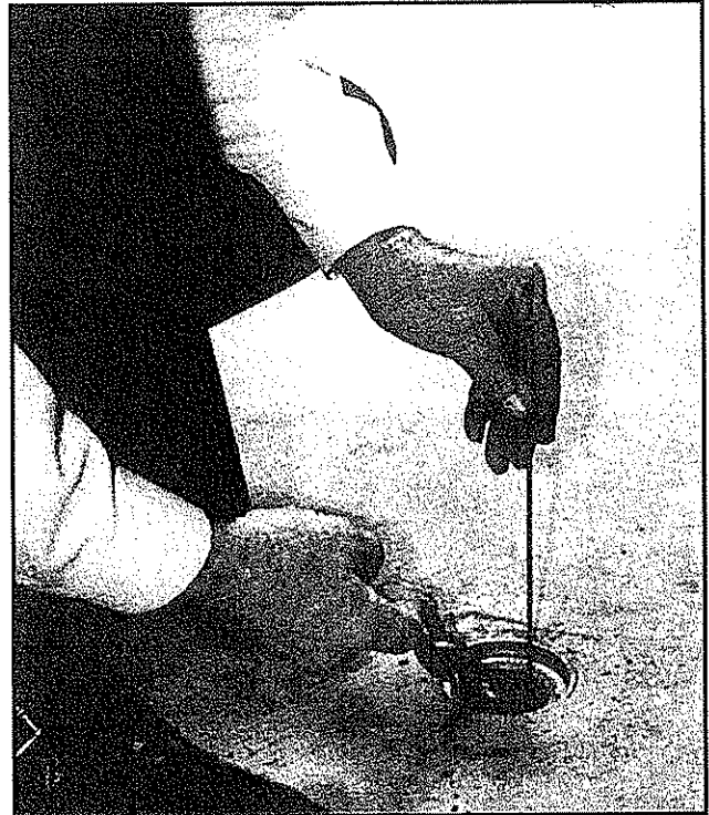
4. Insert hooked end into slot at top of chain retaining wedge.
