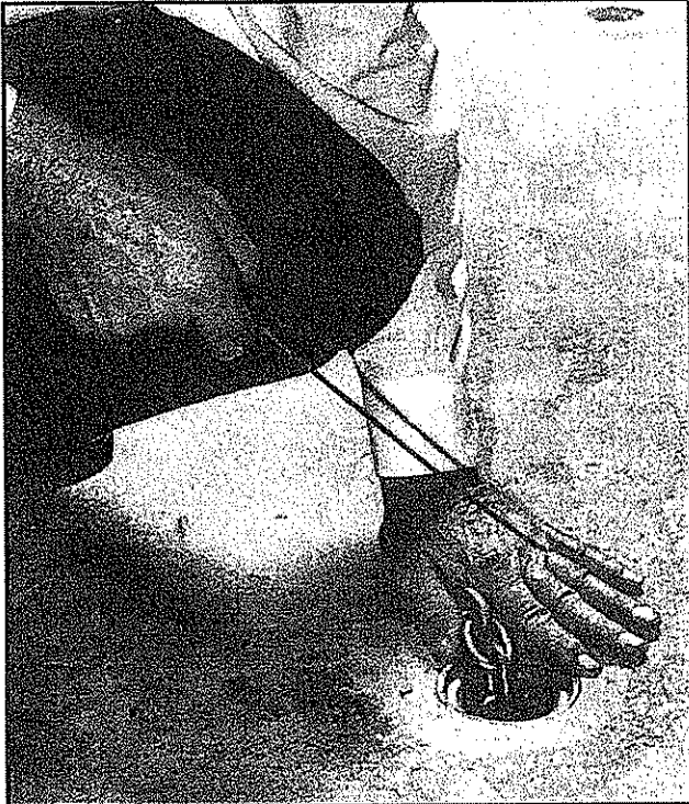
3. Use a length of welding rod with hooked end (or similar tool) as a means to hook into retaining wedge slot.
